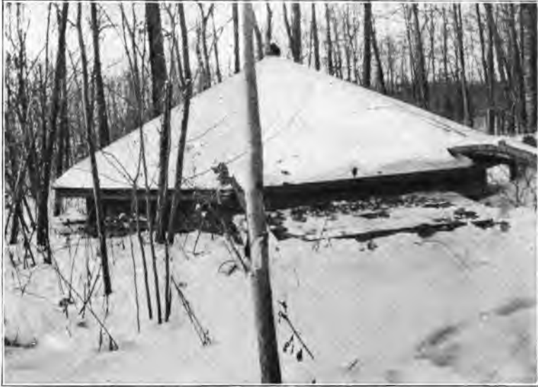
THE LITTLE MUSHROOM-LIKE PUMP HOUSE
